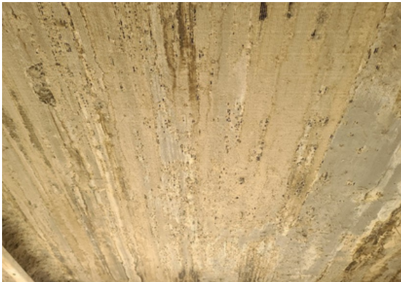
Heat exchanger before dry ice blasting
